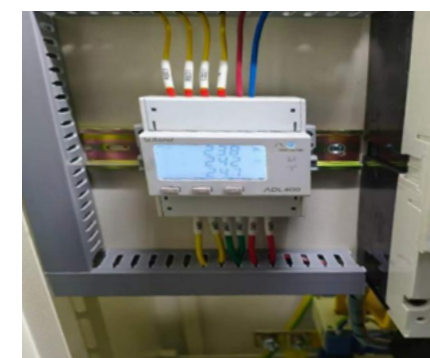
Installation of smart electricity meters
