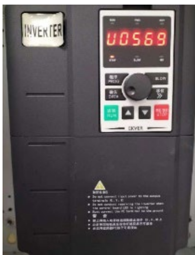
Install frequency converters in SMT air conditioning boxes to reduce power.
