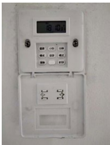
Aisle, bathroom fluorescent lamp, and exhaust fan control time controller
