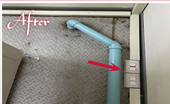
After improvement: The laboratory plugs have been covered with dust-proof covers to reduce the fire risk caused by lint accumulation.
