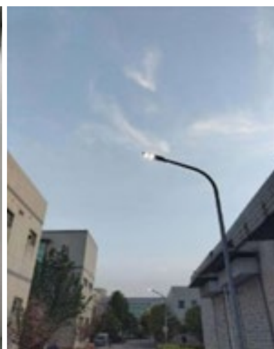
LED lights replace the outdoor street high-pressure sodium lights in the plant area
