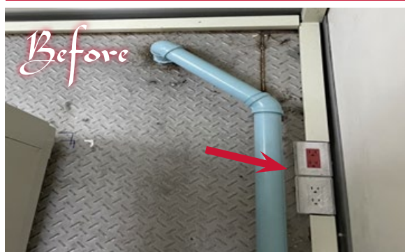
Before improvement: the laboratory plug was not covered with a dust cover
